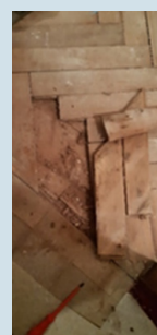
Dismantling test of a wooden floor
