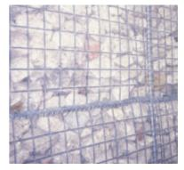
Gabions enable low grade materials to be recycled, but check that wiring will last. Source: F. Stevenson
