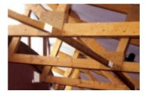
Poorly detailed connectors can prevent effective re-use of timber. Source: F. Stevenson
