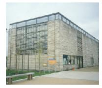
The weathering skin should be removable without damageand disruption to the insulation layer. Source F. Stevenson
