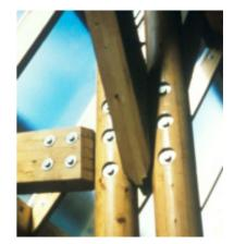
Try to minimise interpenetration of connectors with components. Source: F. Stevenson
