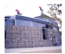
Waste concrete aggregate can be recycled and re-used in numerous ways. Source: F. Stevenson
